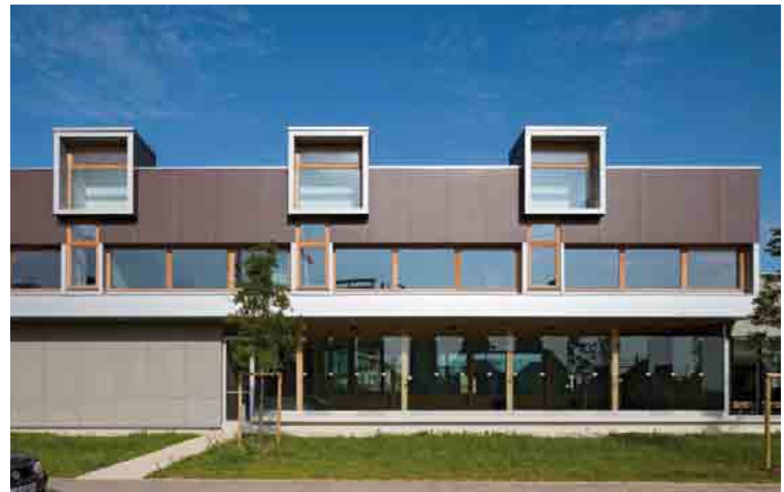
Fibre cement panels in three different colours clad the street façade of the primary school.
