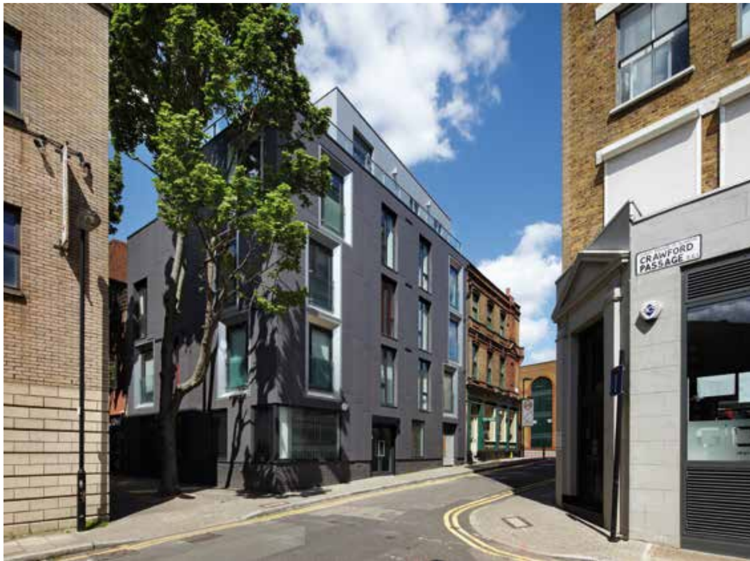
The new corner building fits into the existing building stock like a stone into a mosaic.
