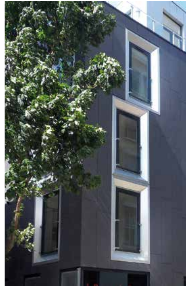
The new façade, with fibre-cement panels staggered in height, and with differently framed French windows.
