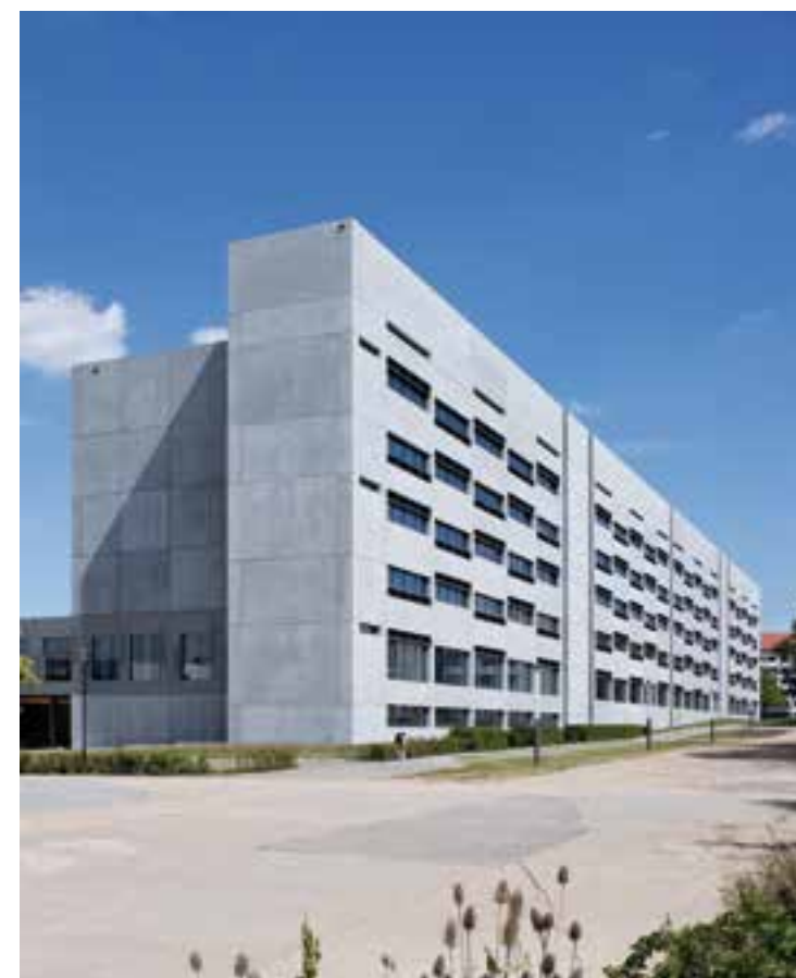
North elevation: Pigmented precast concrete on exterior walls.
