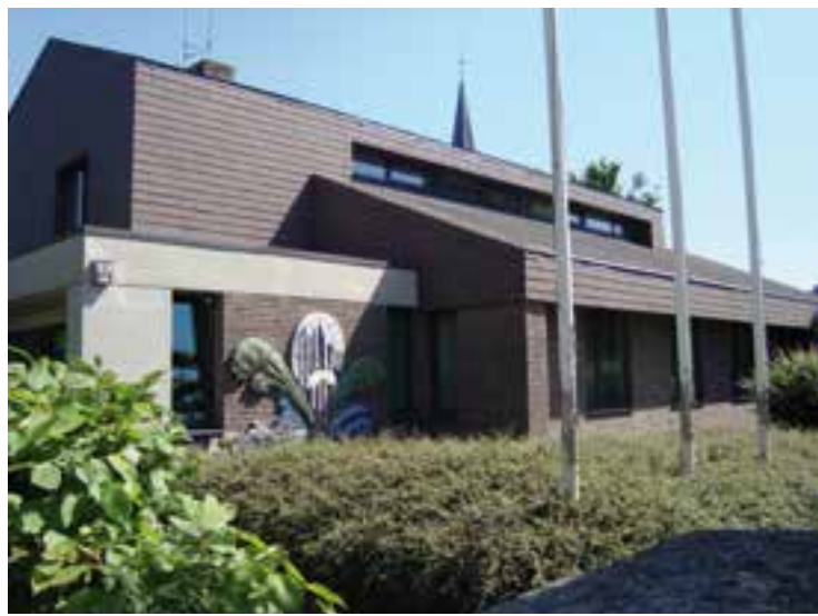
Original structure | Bestandsbau | Existant
