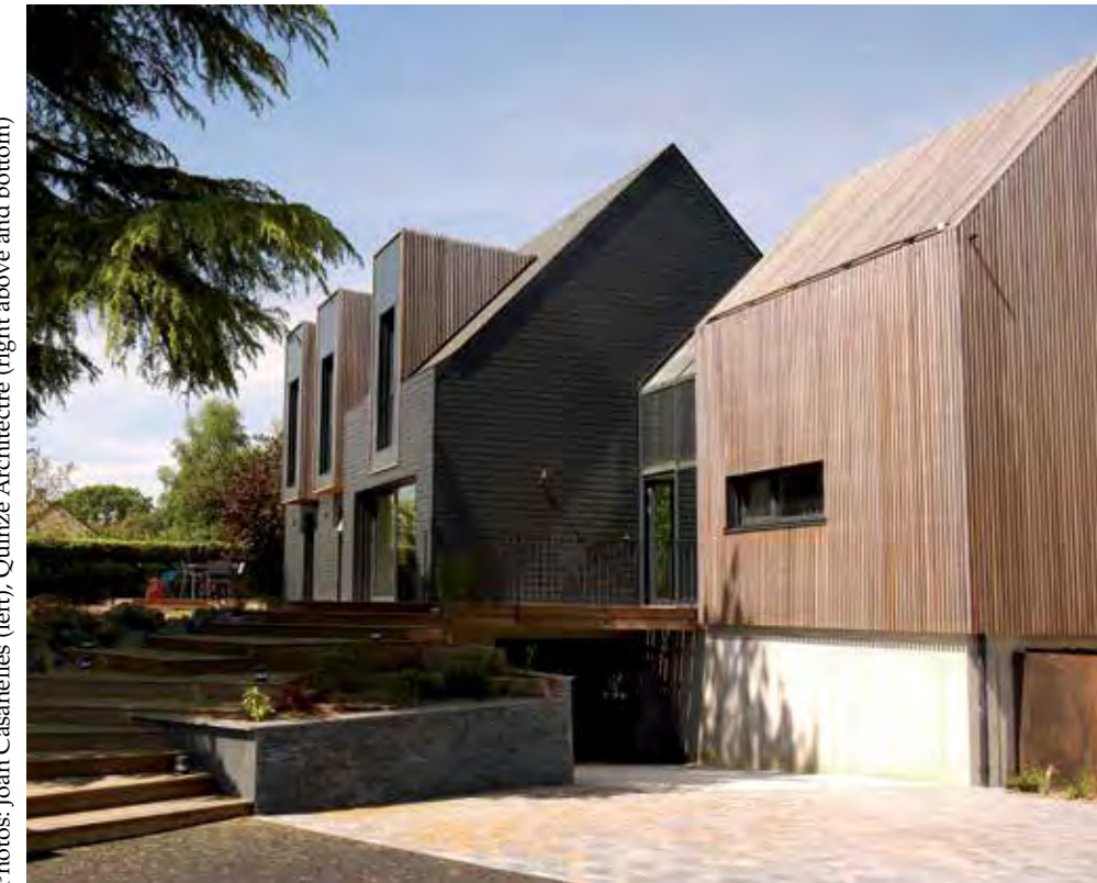
Photos: Joan Casanelles (left), Quinze Architecture (right above and bottom)
