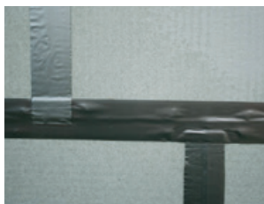
Prinsipp for tapeoverlapping
