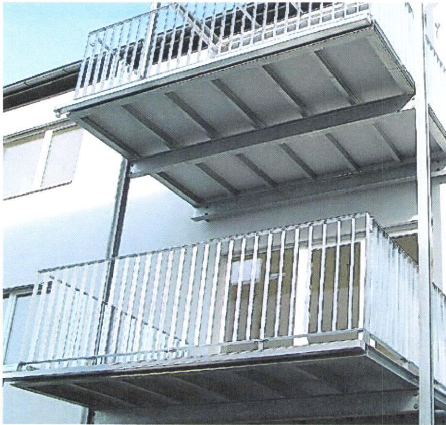
BALCONY FLOOR PANEL SITE IN ST. VEIT/GLAN, AUSTRIA
