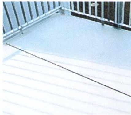
INCLINE AND PANEL JOINTS
